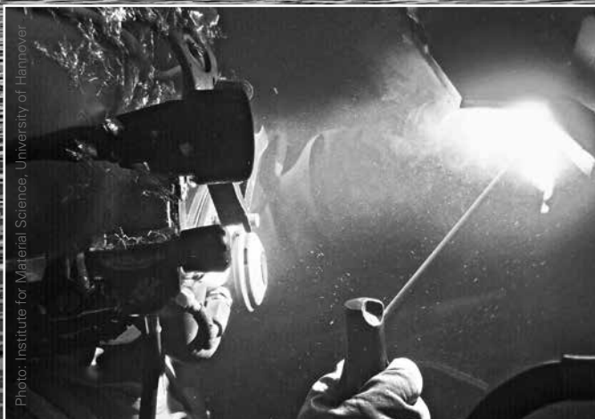
Electric arc welding is still the only process suitable for welding undersea steel structures today.
