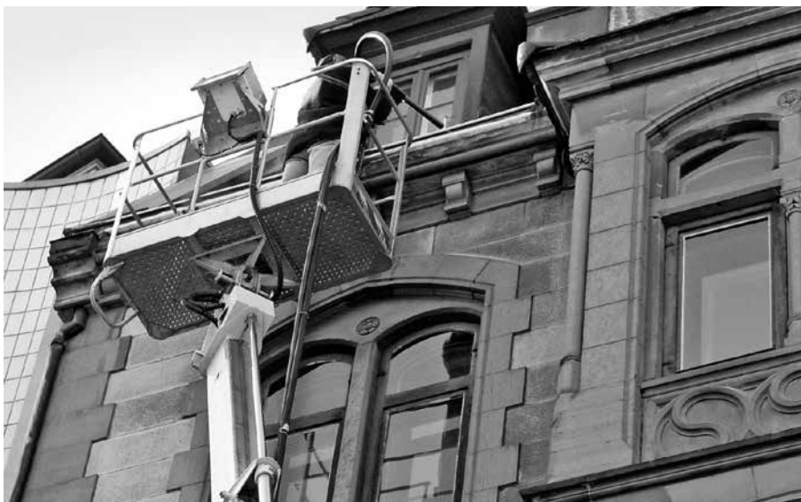
Cleaning with dry ice is gentle on facades and the environment.
