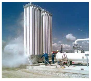
A 70-kilometre section of high-pressure natural gas pipeline was purged with 2,000 cubic metres of nitrogen per hour.
