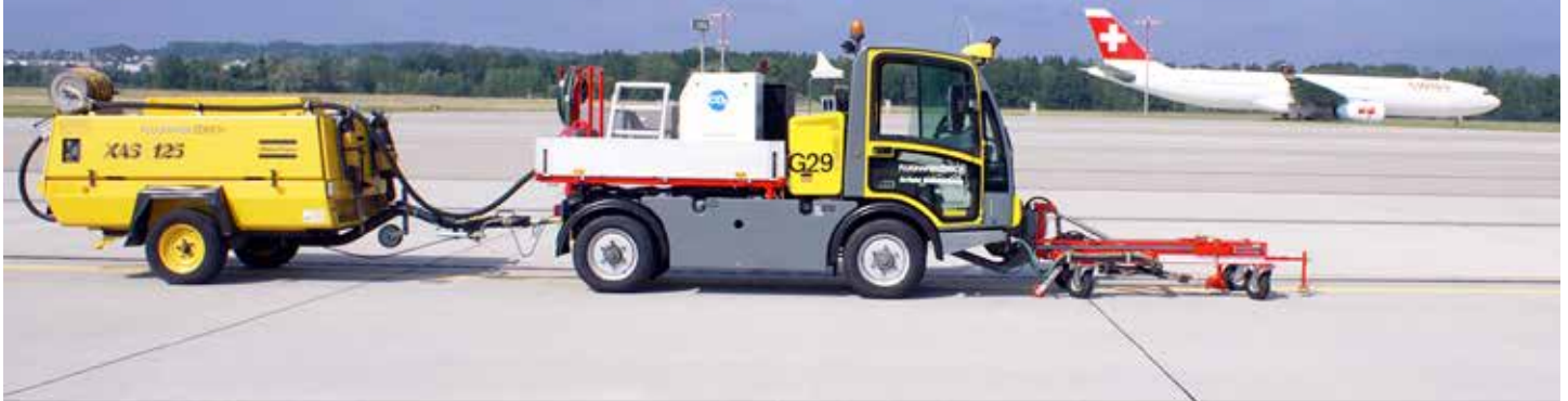
Switzerland: Dry ice blasting at the airport
