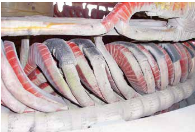
Winding of a power plant generator before and after cleaning with dry ice pellets.
