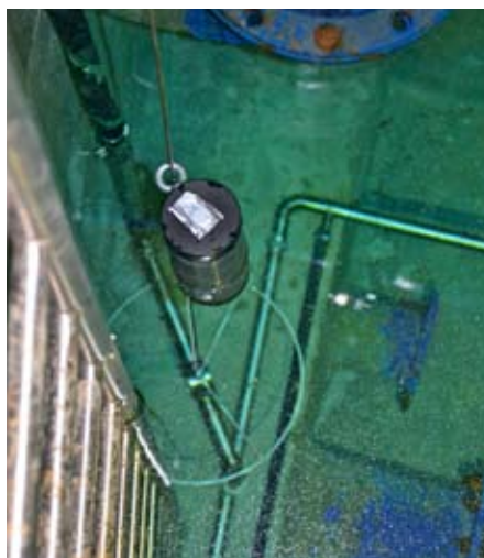
Clearly visible: CO 2 pipes at the bottom of the pump basin
