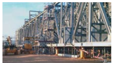
Dismantling a large installation prior to shipping
