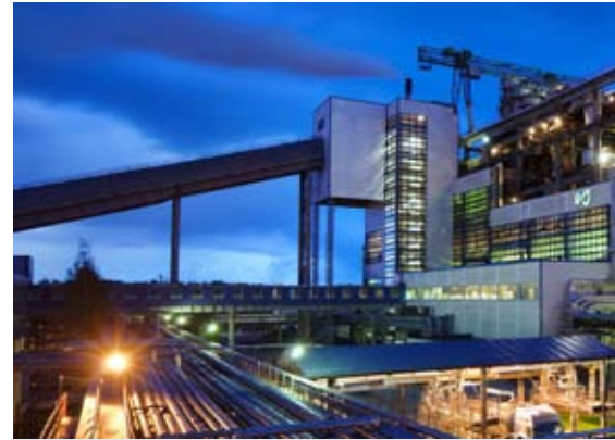
An air separation unit is being built at Eesti Energia
