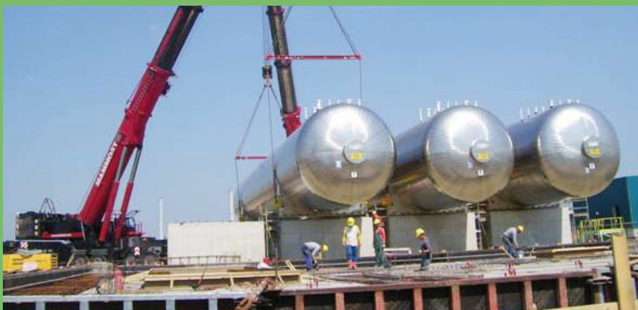
Installation of the storage tanks for the liquefied carbon dioxide
