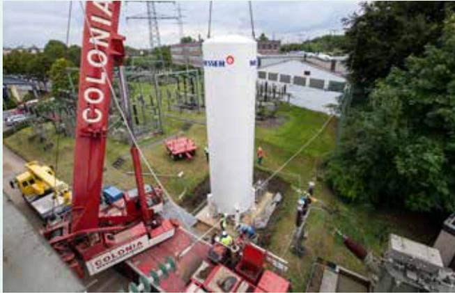
Messer is involved in the development of superconducting power supply cables, which are cooled with liquid nitrogen.
